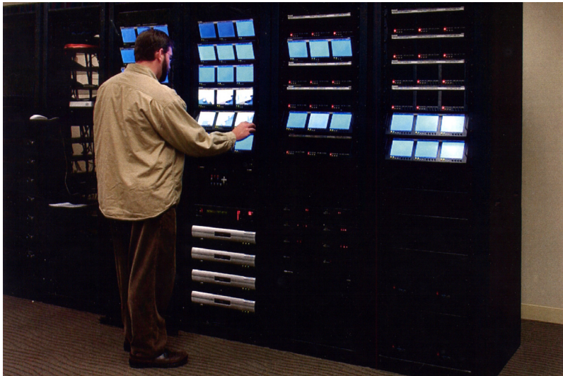
Equipment racks for the Clinical Assessment Center. Each assessment room has its own bank of monitors.
