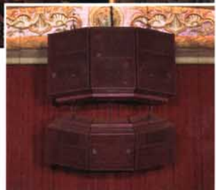
▲ The LARES sound system was designed to blend with the landmark Coronado Theatre in Rockford, IL, avoiding a clash between modern technology and aged architecture. The center cluster consists of EAW AS625, AS660i, AS422 and AS460s.
