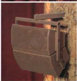
▲ The LARES sound system was designed to blend with the landmark Coronado Theatre in Rockford, IL, avoiding a clash between modern technology and aged architecture. The center cluster consists of EAW AS625, AS660i, AS422 and AS460s.
